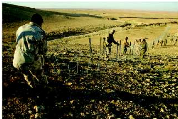
U.S. Marines assigned to 9th Engineer Support Battalion (ESB), 1st Naval Construction Regiment, work with Iraqi Army (IA) soldiers assigned to the 2nd Battalion, 6th Brigade, driving engineer stakes for a wire barrier along the Syrian border in the Ninawa province of Iraq on Dec. 12, 2008.
