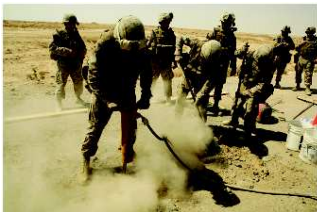
U.S. Marine Lance Cpl. Chris E. Hamrick, a combat engineer 9th Engineer Support Battalion (ESB), 1st Naval Construction Regiment, uses a jackhammer to prepare a pothole for concrete on a road near Lake Habbaniyah in Iraq on September 17, 2008. Part of the mission of 9th ESB during Operation Iraqi Freedom is to improve road conditions for the Iraqi people and coalition forces.
