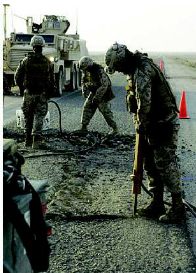
U.S. Marine Lance Cpl. Cody D. Locklear, a combat engineer 9th Engineer Support Battalion (ESB), 1st Naval Construction Regiment, uses a jackhammer to prepare a pothole for concrete on a road near Lake Habbaniyah in Iraq on September 17, 2008. Part of the mission of 9th ESB during Operation Iraqi Freedom is to improve road conditions for the Iraqi people and coalition forces.
