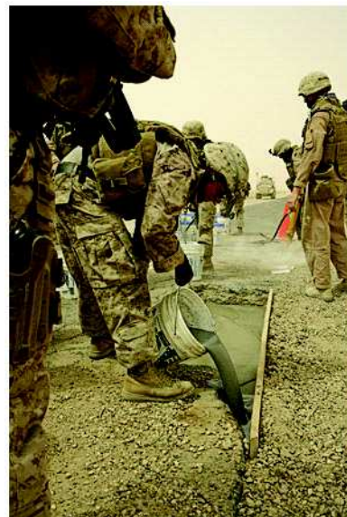
U.S. Marine Lance Corporal Adam T. Derr, a combat engineer with 9th Engineer Support Battalion (ESB), 1st Naval Construction Regiment, pours concrete into a pothole on a road near Taqaddum, Iraq on September 10, 2008. Part of the mission of 9th ESB during Operation Iraqi Freedom is to improve road conditions for coalition forces as well as the Iraqi people.
