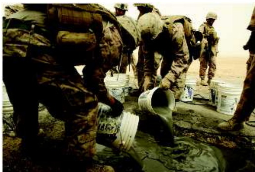
U.S. Marine Corporal Robert C. Knudson, right, and Lance Corporal Adam T. Derr, both with 9th Engineer Support Battalion (ESB), 1st Naval Construction Regiment, pour concrete into potholes on a road near Taqaddum, Iraq on September 10, 2008. Part of the mission of 9th ESB during Operation Iraqi Freedom is to improve road conditions for coalition forces as well as the Iraqi people.
