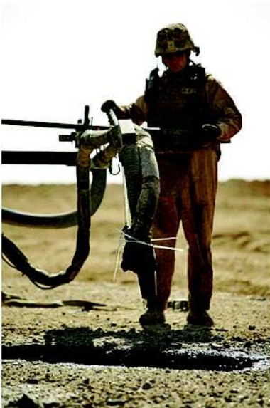
U.S. Marine Cpl. Richard House, a combat engineer from Toledo, Ohio, assigned to 9th Engineer Support Battalion (ESB), 1st Naval Construction Regiment, fills a hole using a magnum spray injection patcher during a route repair mission near Lake Habbaniyah on Nov. 1, 2008. Part of 9th ESB's mission during Operation Iraqi Freedom is to improve road conditions for the Iraqi people and coalition forces.
