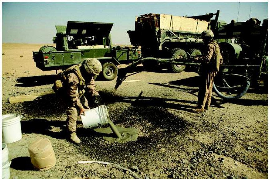
U.S. Marines Lance Cpl. Ray Foronda, left, and Cpl. Richard House, assigned to 9th Engineer Support Battalion (ESB), 1st Naval Construction Regiment, repair a hole during a route repair mission near Lake Habbaniyah on Nov. 1, 2008. Part of 9th ESB's mission during Operation Iraqi Freedom is to improve road conditions for the Iraqi people and coalition forces.
