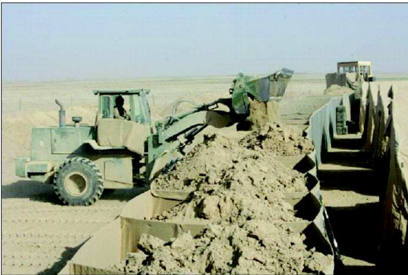
A CLB-3 TRAM hard at work filling HESCO at a Combat Outpost.
