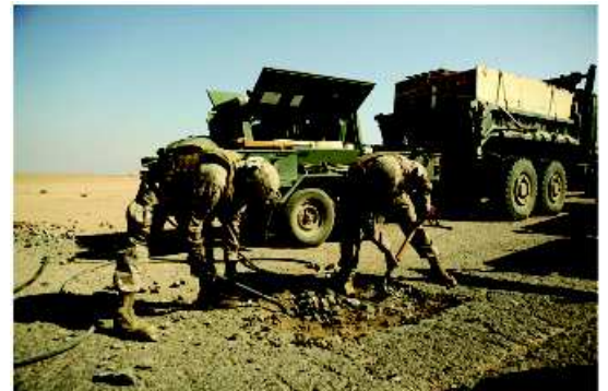
U.S. Marine Gunnery Sgt. Karleton Lawrence, left, and Staff Sgt. Fred Maldonado, assigned to 9th Engineer Support Battalion (ESB), 1st Naval Construction Regiment, remove broken concrete from hole during a route repair mission near Lake Habbaniyah on Nov. 1, 2008. Part of 9th ESB's mission during Operation Iraqi Freedom is to improve road conditions for the Iraqi people and coalition forces.
