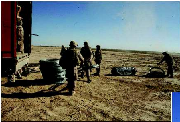
Engineers offload concertina wire to construct an antipersonnel fence at a Combat Outpost in Afghanistan. An infantryman stands post after CLB-3 Engineers constructed a guard tower.
